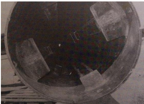
Figure 4-31 Bottom of Toe Section. Channel covers are clearly visible, Cox et al. (1992).
